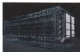
18 Holland Park School London, England. Architect: Aedas
