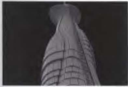
8 K. Çamlica TV Tower Istanbul, Turkey. Architect: Melike Altinisik
